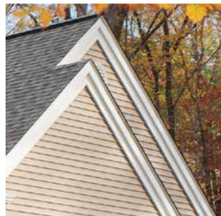
5" Trimworks lineals used as "rake" boards.
